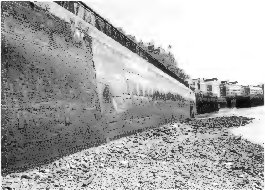
FIGURE 7. Near-vertical river wall at Wapping; the brick wall in the foreground is covered by green algae while the concrete wall in the background has a less-extensive cover, May 2012.
